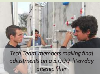
Working on phase one of our first Groundwater Treatment System
